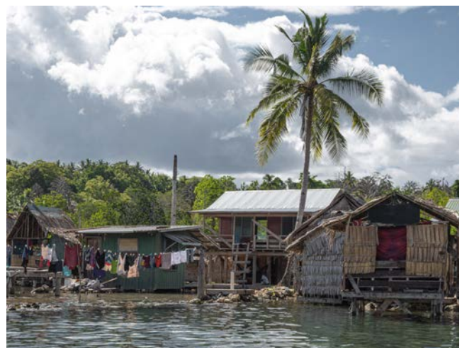
Nsugaraku, one of the villages affected by rising sea levels
